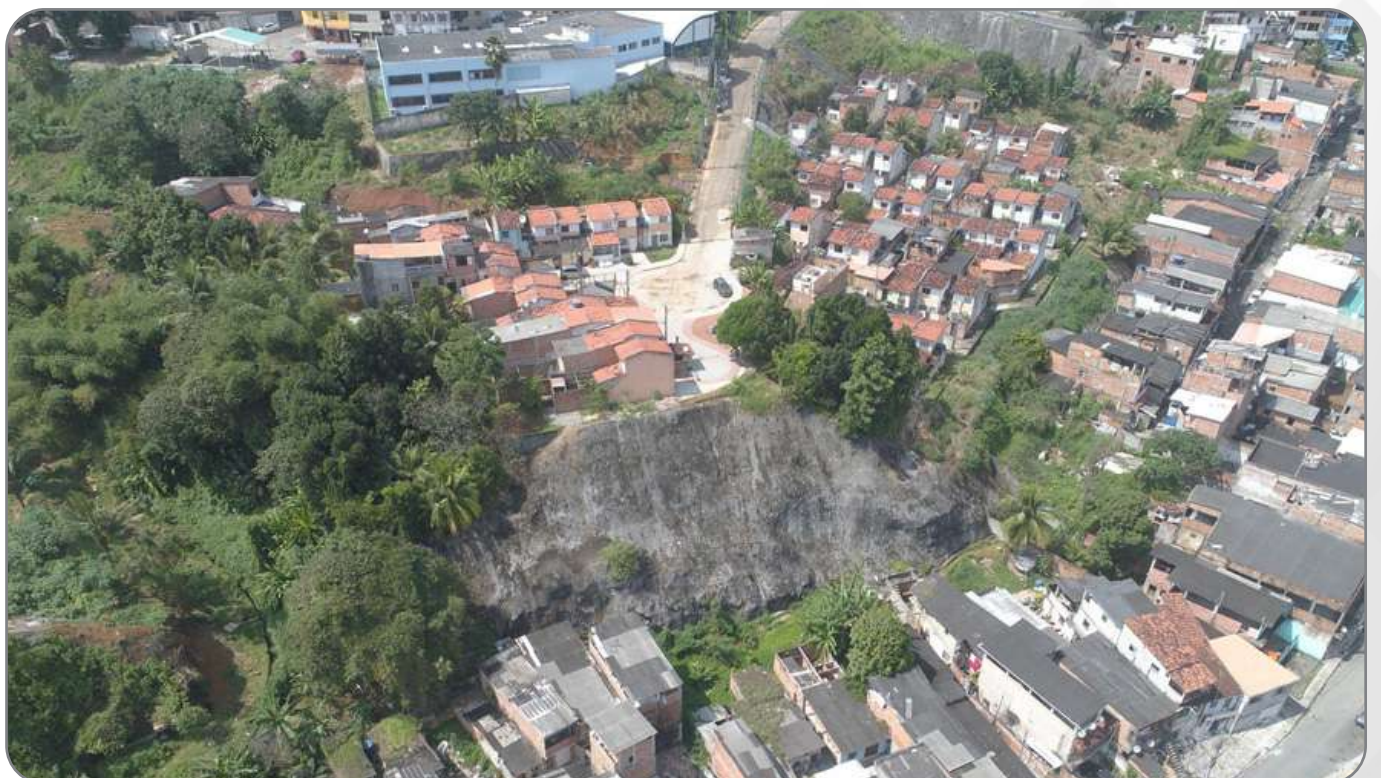
Slope Containment and Slum Urbanization at PDE 124
