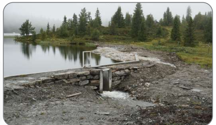
The old stone masonry dam from 1870 at Lake Svintjønnå before revitalization.
