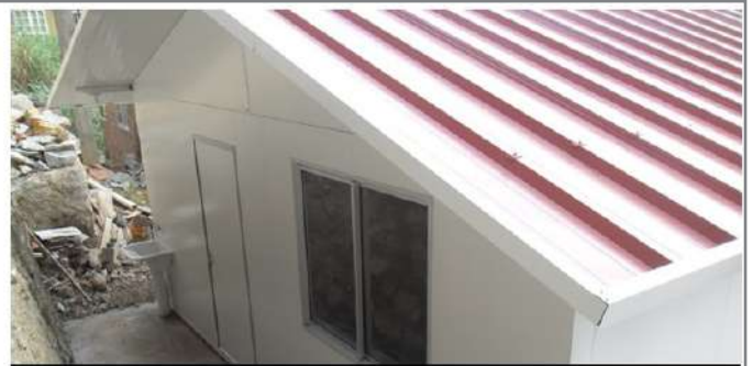
Modular House at Morro do Céu Community
