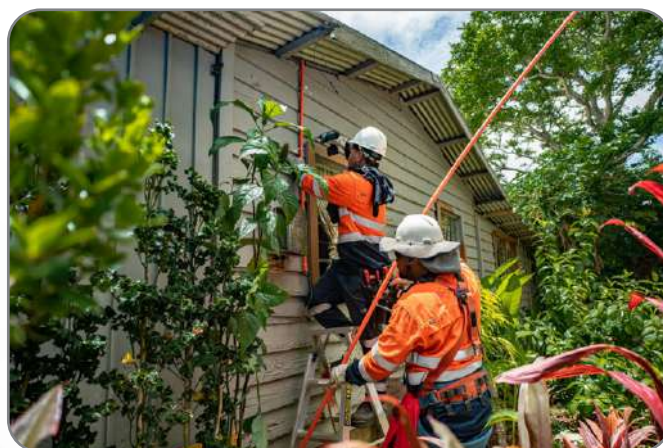
Installation of electric conduits on building walls
