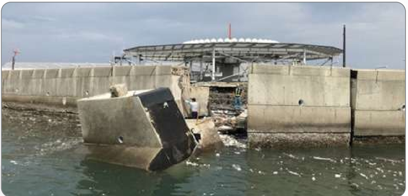
Disaster countermeasures being installed at Kansai International Airport after typhoon on 4th September, 2018
