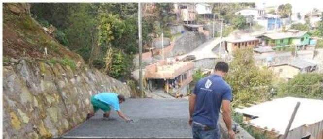
Paving in Caiera Community
