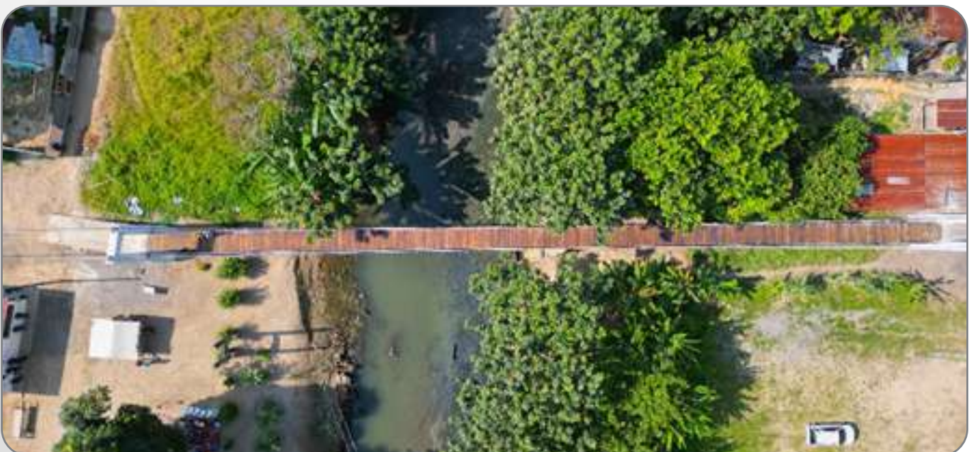
The pedestrian bridge on Roberto Luis Cervantes Island connects the island with the mainland
