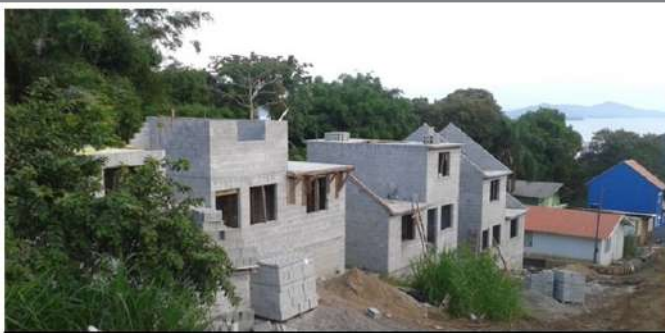
Structural Masonry House at Nova Descoberta Community
