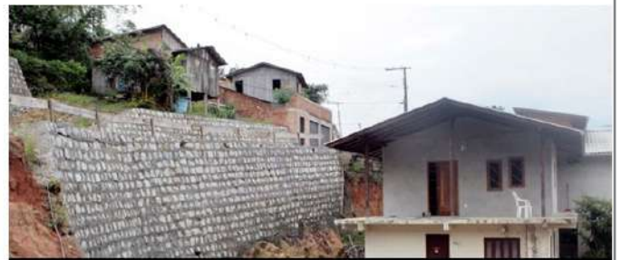
Slope Containment at Caiera Community
