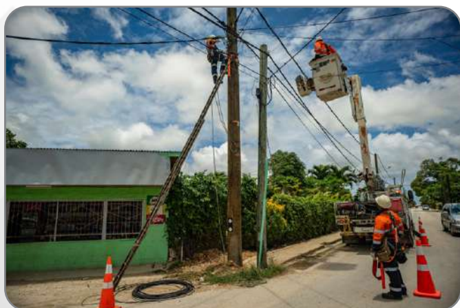
Maintenance activities of energy infrastructure in Tonga
