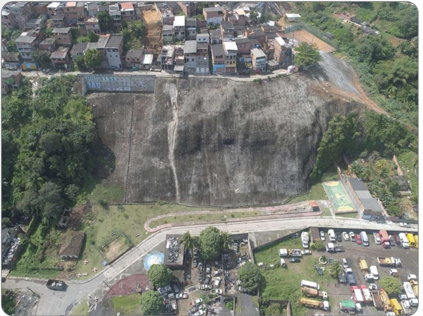
Slope Containment and Slum Urbanization at PDE 124
