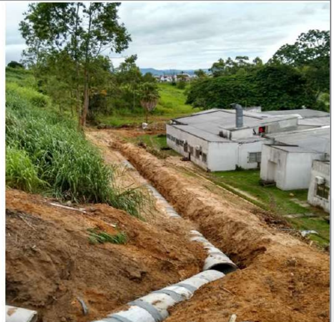
Drainage System at Santa Vitoria Community
