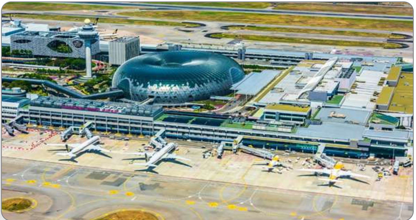
Changi Airport Source: Royal HaskoningDHV
