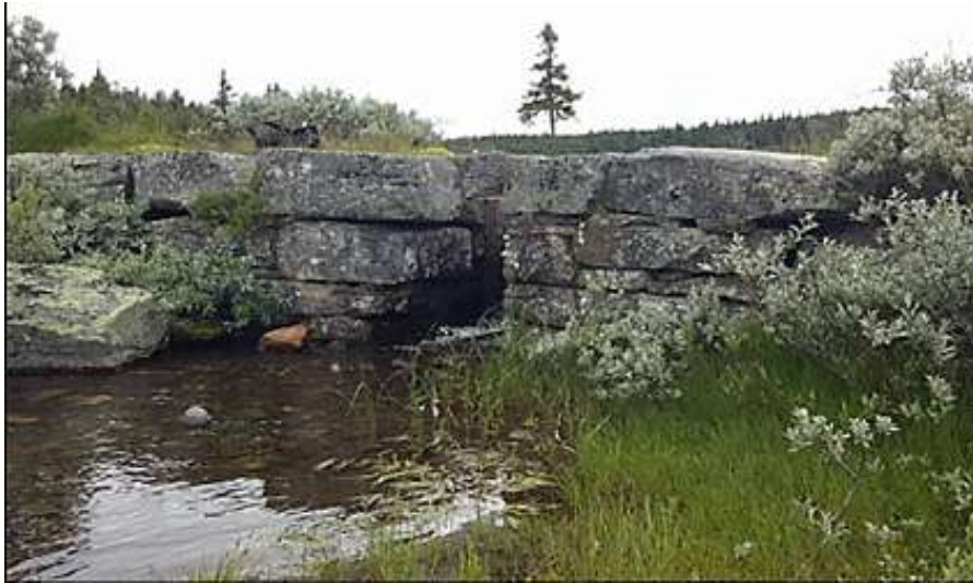
The old stone masonry dam from 1870 at Lake Svintjøna before revitalization.
